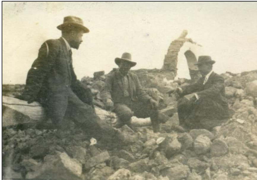
141 Caption beneath picture says, "Shattered by a Shell."
