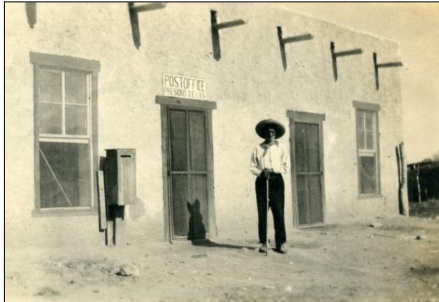
014 Labeled, "La Botica." Sign over door says "Post Office, Presidio, Texas."
