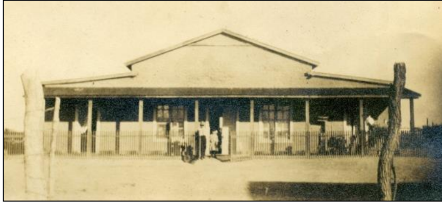
012 Unlabeled. Building must be in or around Presidio.
